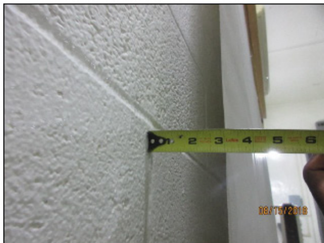
Photo No. 2 Side View of Installed Specimen
